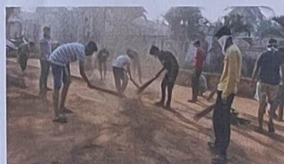
Cleaning of roads
