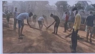
Cleaning of roads
